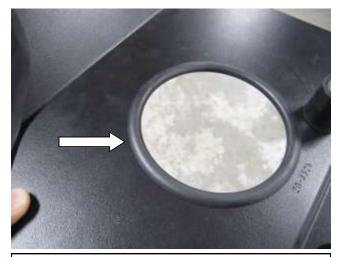
e. Install the supplied edge trim (102466) onto the inner part of the heat shield.
