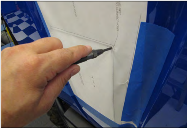
13. Mark the hole locations in each corner using a center punch.
