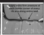
Continue around corner . At floor, leave protective backing to wall side. Work across floor with firm pressure up and down each rib. Then peel backing off wall side and apply pressure to it. Next continue with both seals up box. Stop at box contour near top. Leave adhesive protectors on- mark and cut seal to length for top and V-cut - as at top of other side -then finish adhering.
