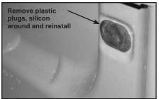
b) Black nylon wall plugs. Seal if desired c) by removing each one applying silicon around perimeter and reinstalling.
