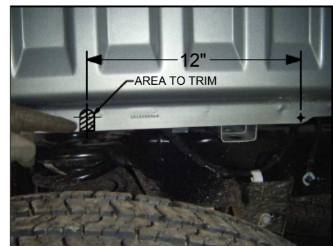
Figure 10.1: Inside Driver Side Rear Wheel Well
