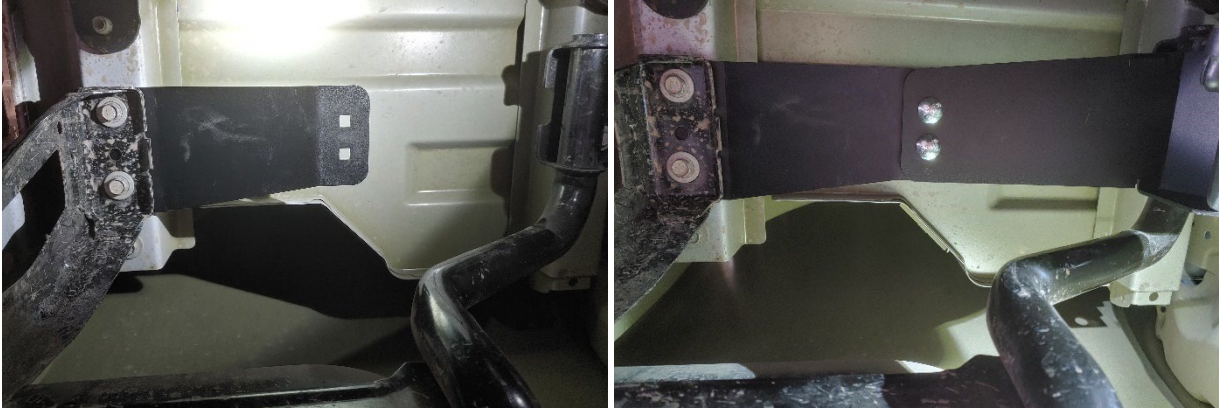
Figure 21- Passenger Side Bracket Install, Brackets Temporarily Secured
