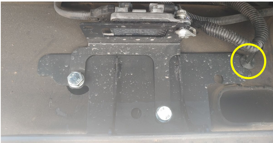
Figure 36- Compressor Bracket Installation 2, Diesel
